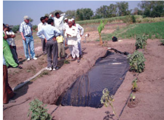
Example of a small water storage trench in India
